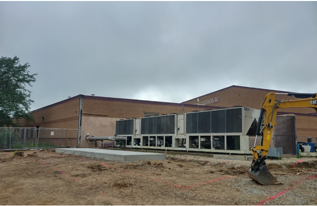
Concrete pad for new chiller
